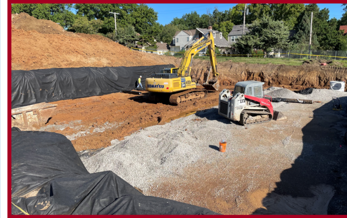
Underground Detention Basin Excavation
