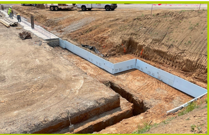
CIP Retaining Wall Footings
