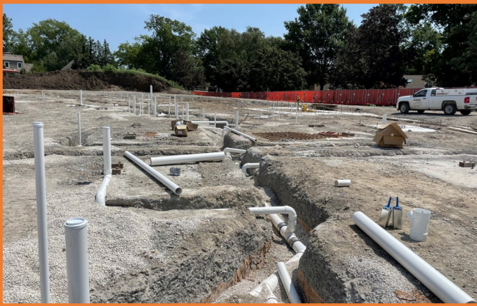
Classroom Wing Underground Plumbing
