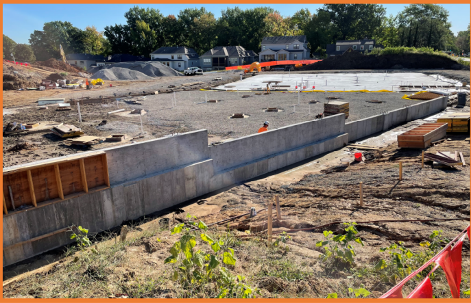
Classroom Wing - Retaining Wall Pours
