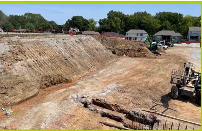
Gym CIP Footing Excavation
