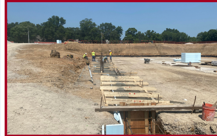
Area C Classroom Wing Grade Beams
