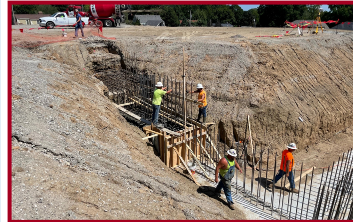
Gymnasium - Footing Reinforcement
