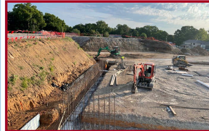
Classroom Wing CIP Retaining Wall Footings
