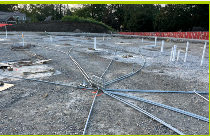
Classroom Wing Underslab Electrical
