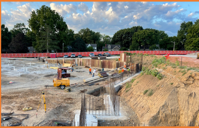
Classroom Wing CIP Wall Reinforcing
