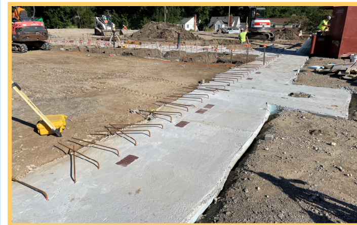
Gym Footings & Precast Embed Plates
