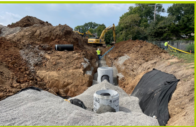
Underground Storm Sewer Piping
