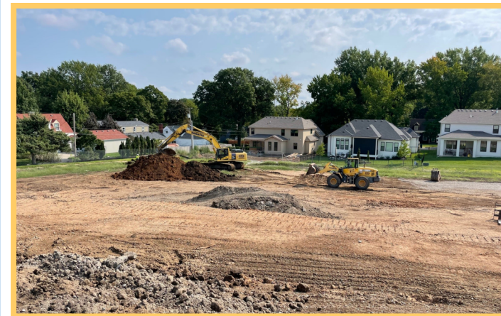
Underground Detention Excavation
