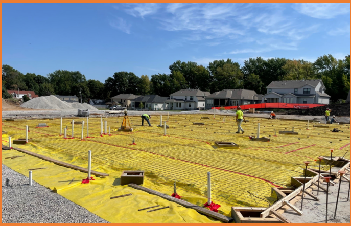
Classroom Wing - Slab-on-Grade Prep
