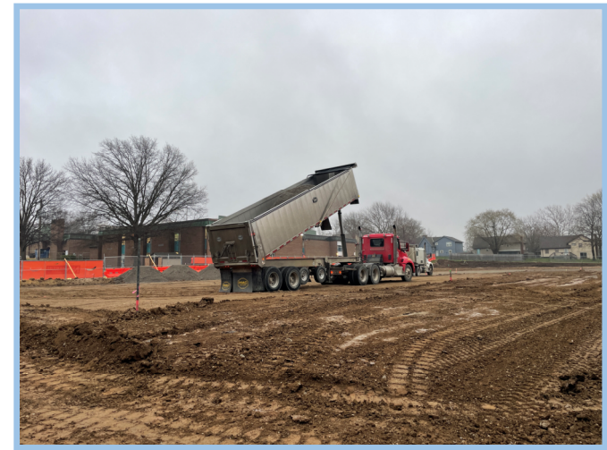
Imported Material For Building Pad
