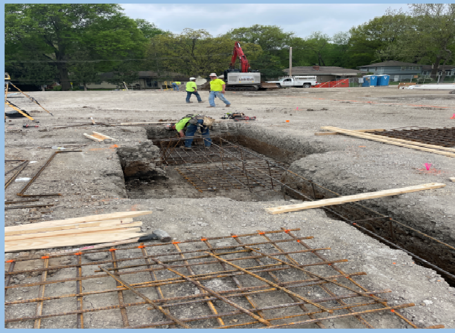
Footing Reinforcement Install
