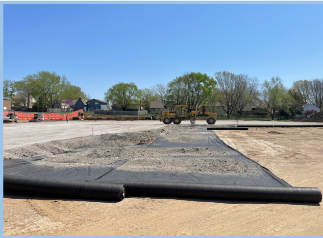
Laydown Filter Fabric
