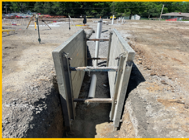
Plumbing Underground Sanitary
