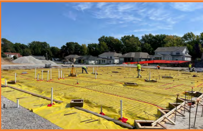
Classroom Wing - Slab-on-Grade Prep
