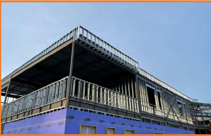
Area C - Exterior / Parapet Framing
