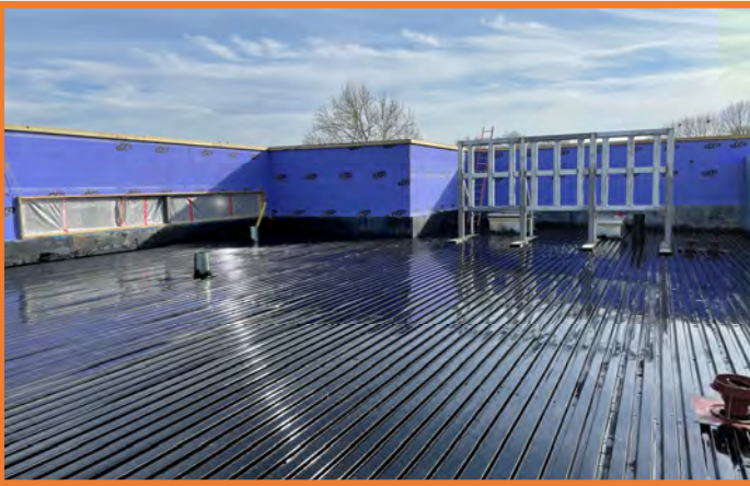
Area B & A Roof - Primed & Insulated
