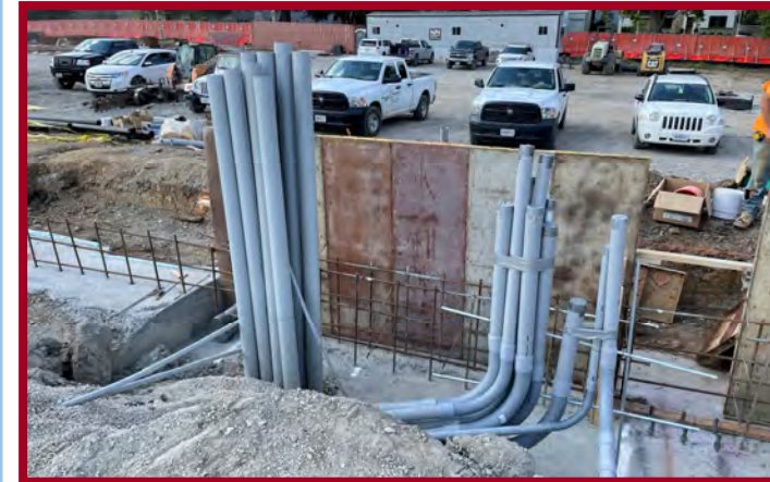
Electrical Service - Building Entry Conduits
