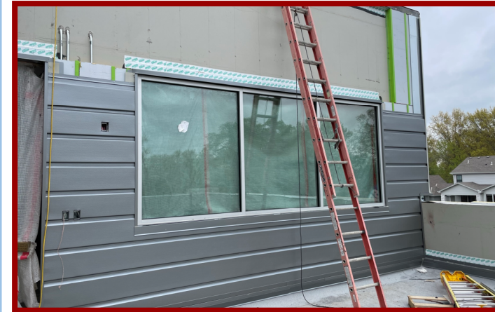
Continued Metal Panel Installation
