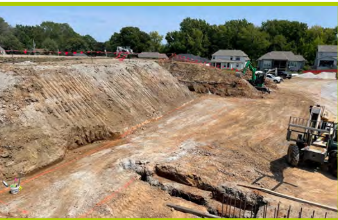
Gym CIP Footing Excavation
