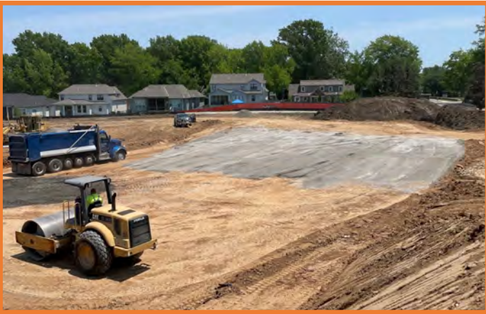
Building Pad Installation
