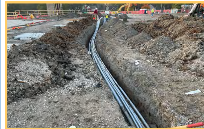
Area B Underground Electrical
