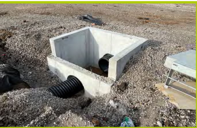
Storm Sewer Piping & Inlets
