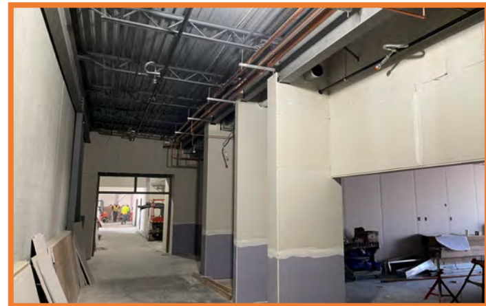
Area A Drywall Finishing
