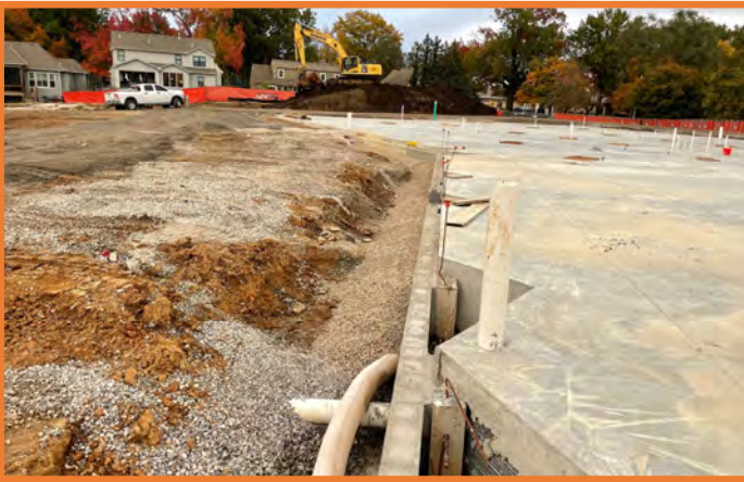
Area C Foundation Drainage & Backfill
