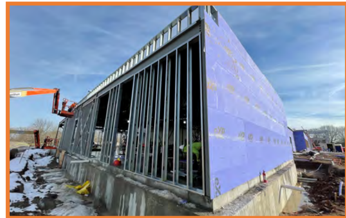
Area A - Exterior Framing & Sheathing
