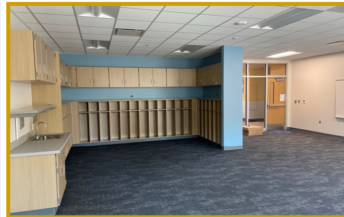
Ceiling Tile & Rubber Base Installed
