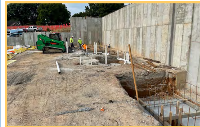
Elevator Pit Footing & Underslab Plumb.
