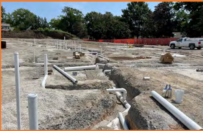
Classroom Wing Underground Plumbing
