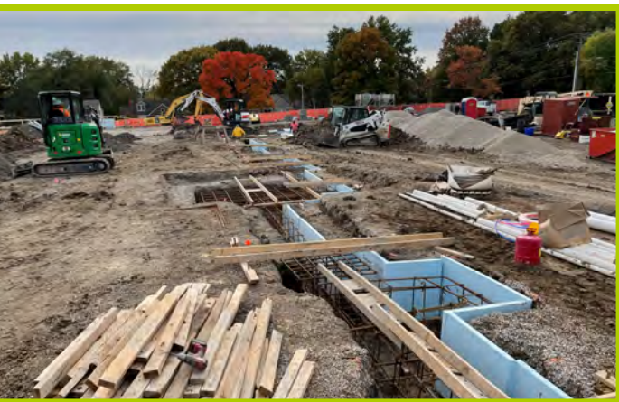
Area B Grade Beam Reinforcement
