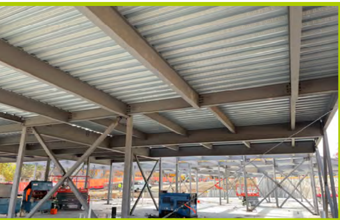
Area C 2nd Floor Metal Decking
