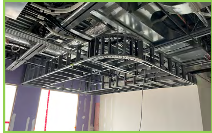
Reception Soffit Framing
