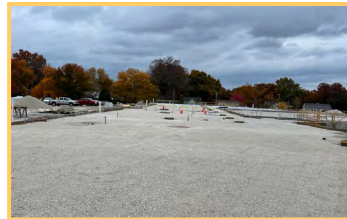
Area B Slab-on-Grade Prep
