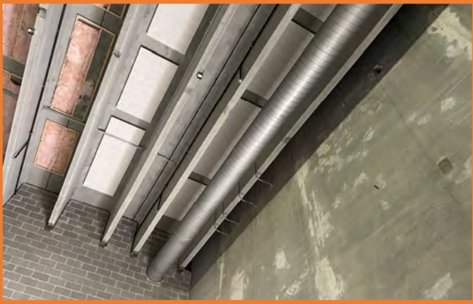
Gym Ductwork and Ceiling Tectum Panels
