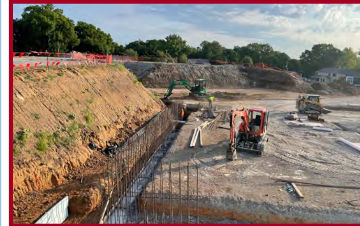
Classroom Wing CIP Retaining Wall Footings
