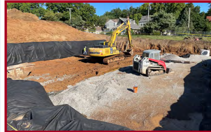
Underground Detention Basin Excavation
