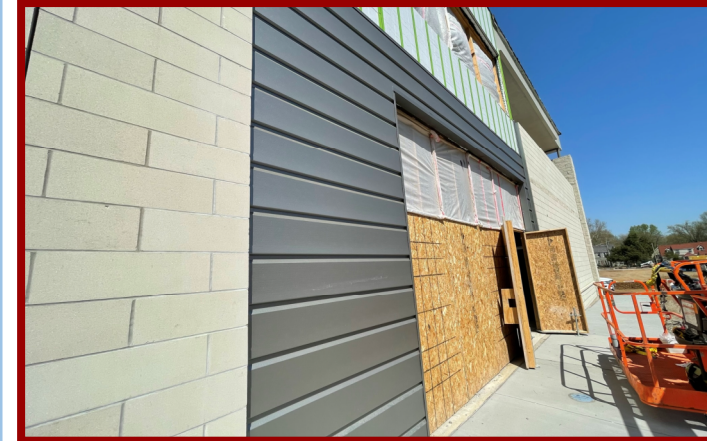
Metal Panel Installation
