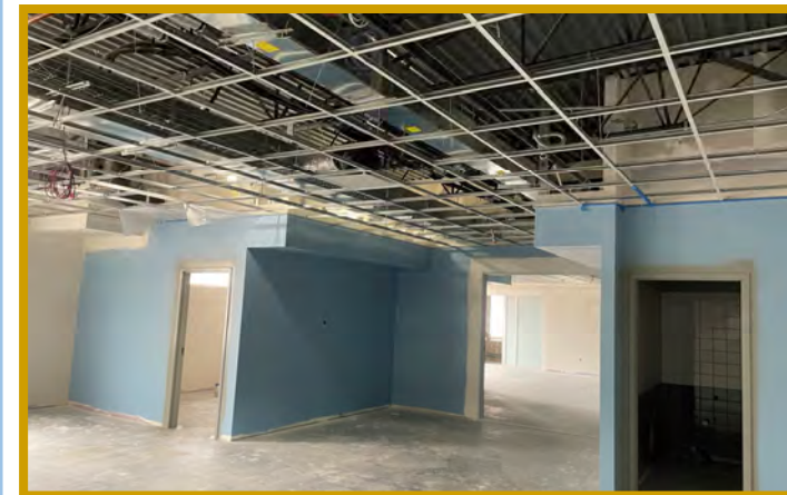
Upper Level Ceiling Grid & Paint
