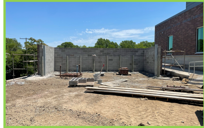
Trash Enclosure CMU & Brick Veneer
