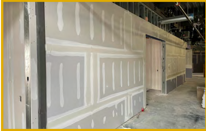
Area C Lower Level Drywall Tape & Finish
