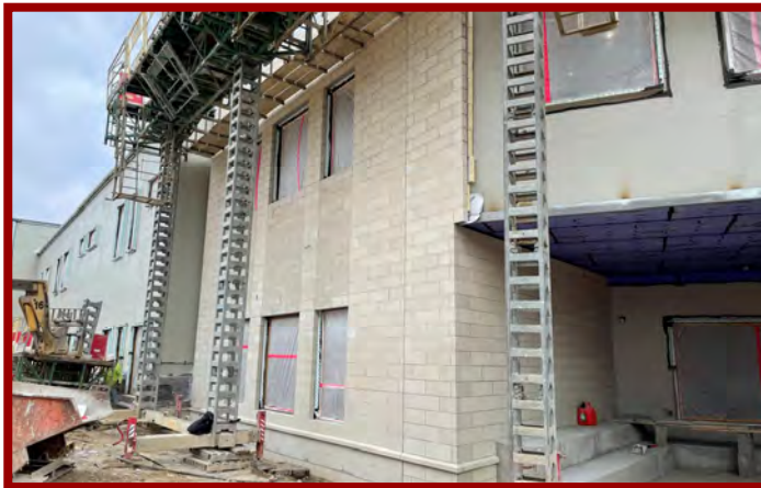
Area C Masonry Veneer Progress
