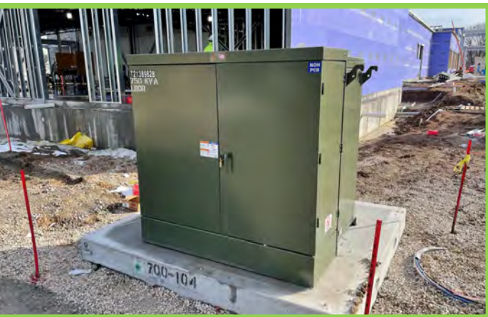
Transformer Set & Temp Power Running
