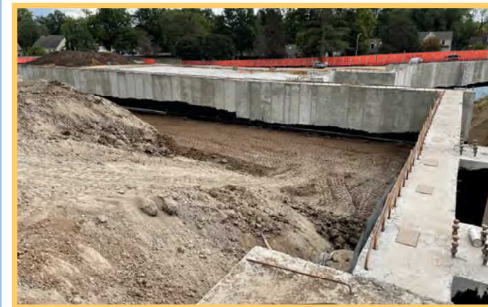
Gym Retaining Wall - Interior Backfill
