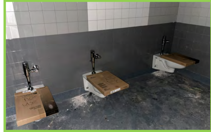
Lower Level Plumbing Fixture Install
