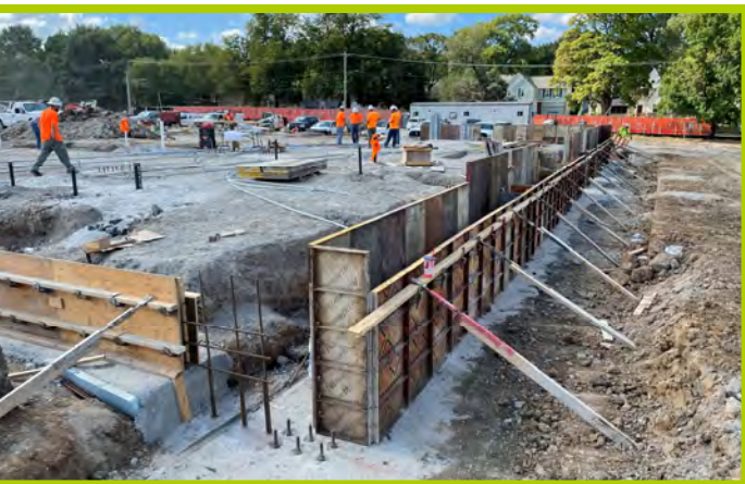
Area A - Stem Wall Formwork & Pours
