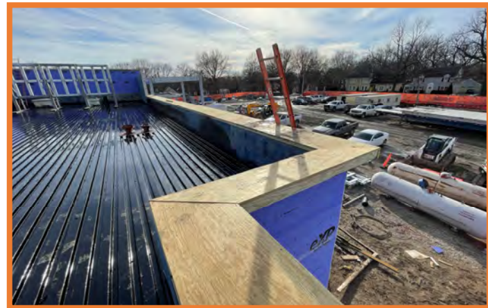
Area A Continued Parapet Blocking
