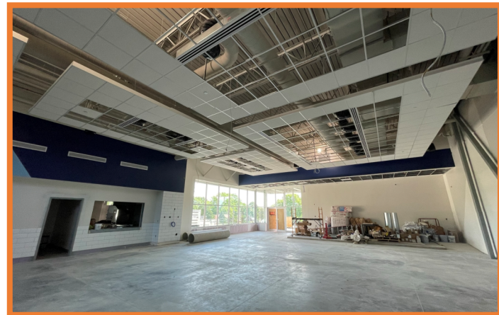
Commons Area Polished Concrete Grinding
