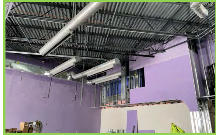
Media Center - Soffit Framing & Drywall Hang
