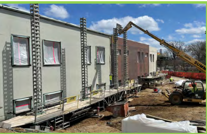
Area C Masonry Veneer Progress
