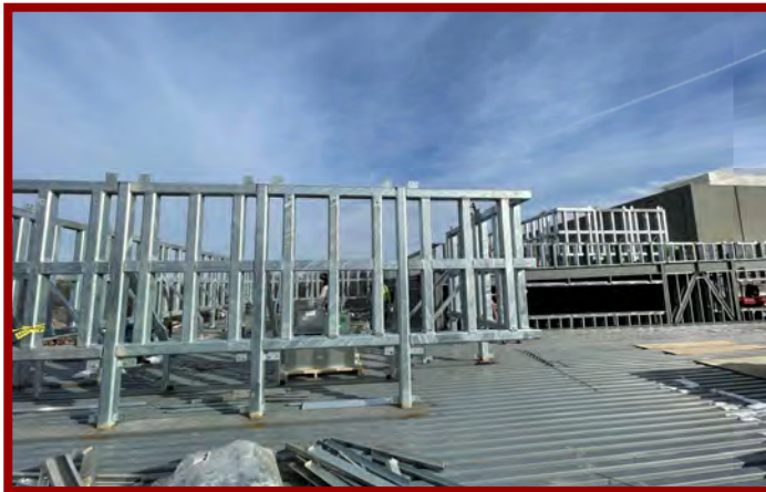
Area A - RTU Screen Framing
