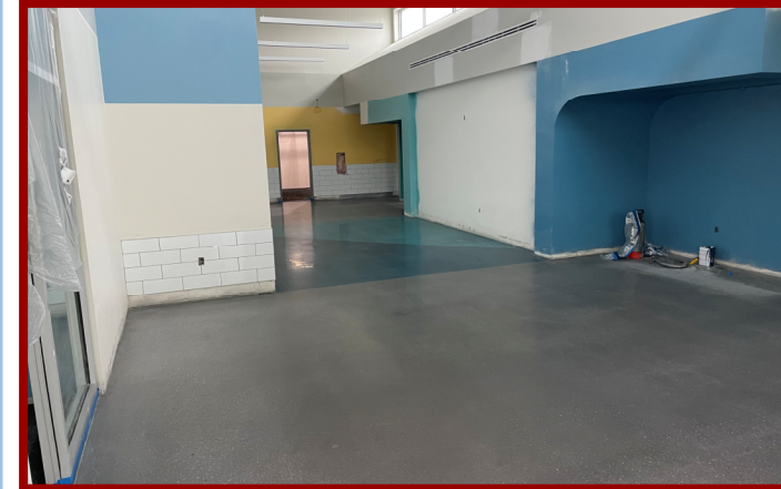
Polished Concrete - Staining & Sealing
