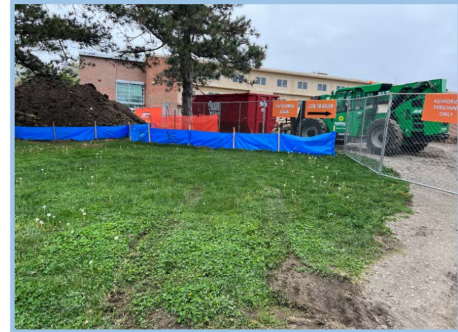
Added SWPP Around Stock Pile
