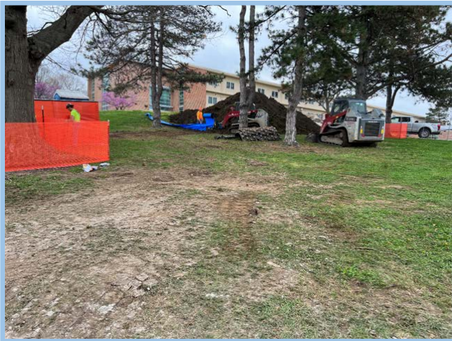
Erosion Control & Tree Protection
