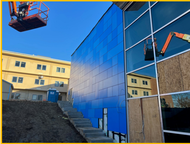
North Elevation Phenolic Panel
