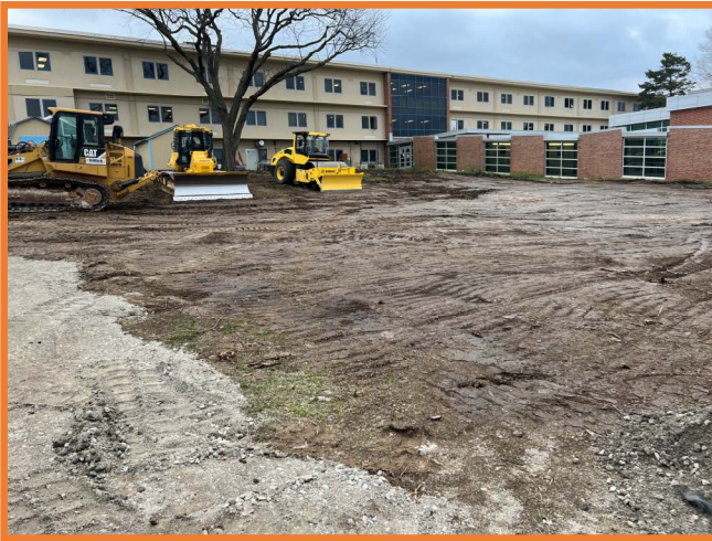
Site Clearing & Grading
