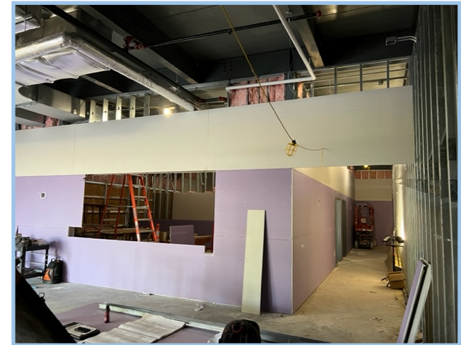
Level 3 Drywall Hang & Finish
