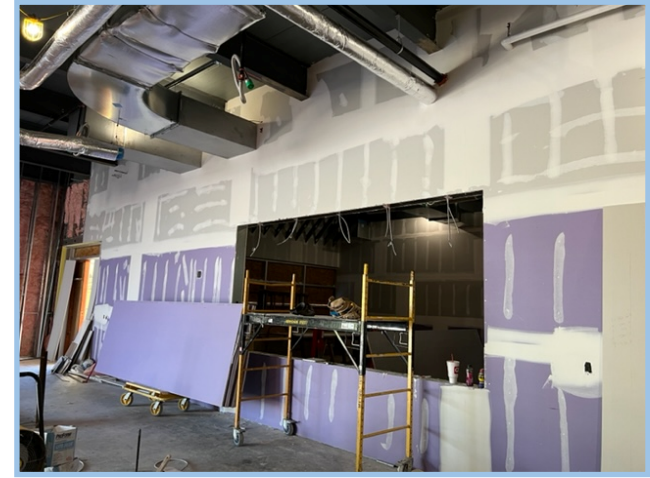
Level 3 Drywall Tape & Finish
