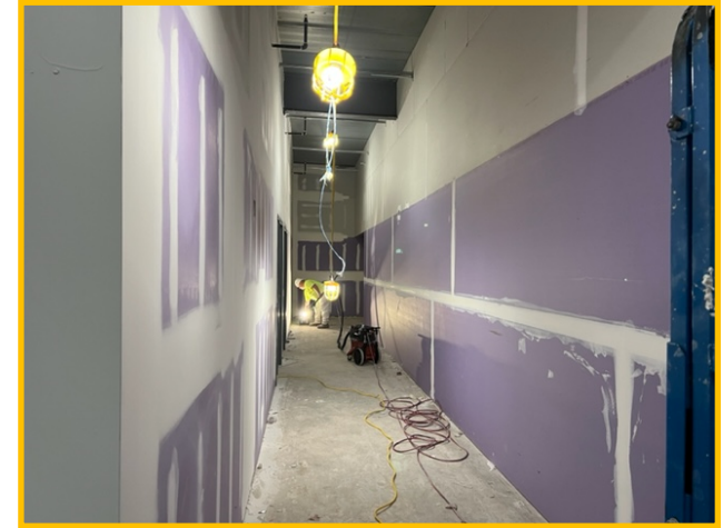
Level 3 Drywall Tape & Finish
