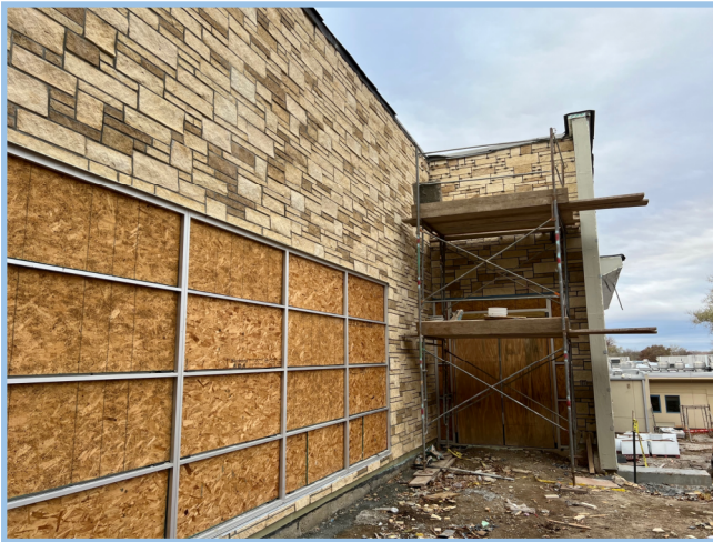
North Elevation Stone Veneer
