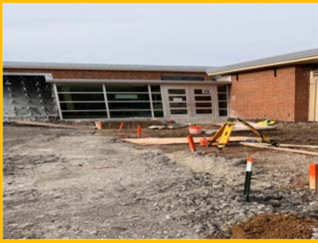
Layout Footings & Foundations
