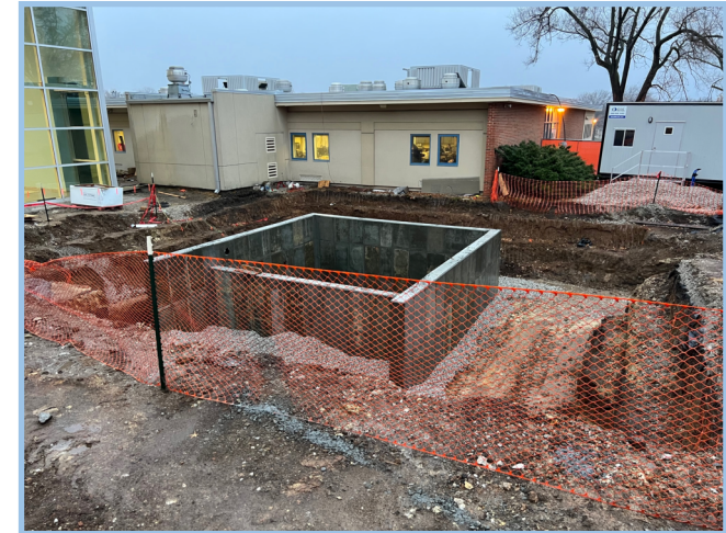
Courtyard Detention Basin Backfill
