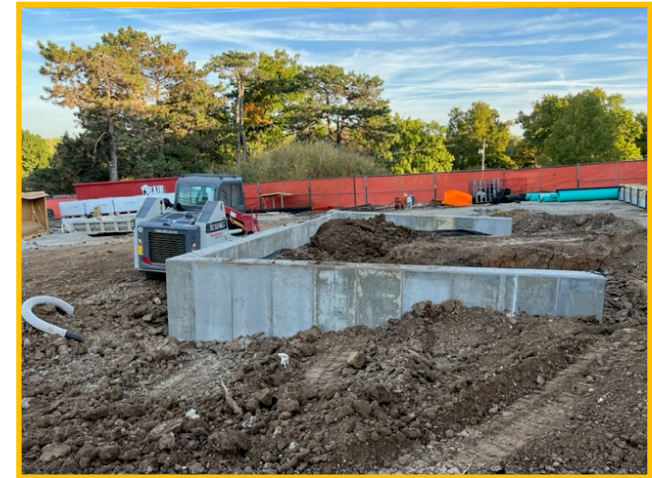
Courtyard CIP Retaining Walls
