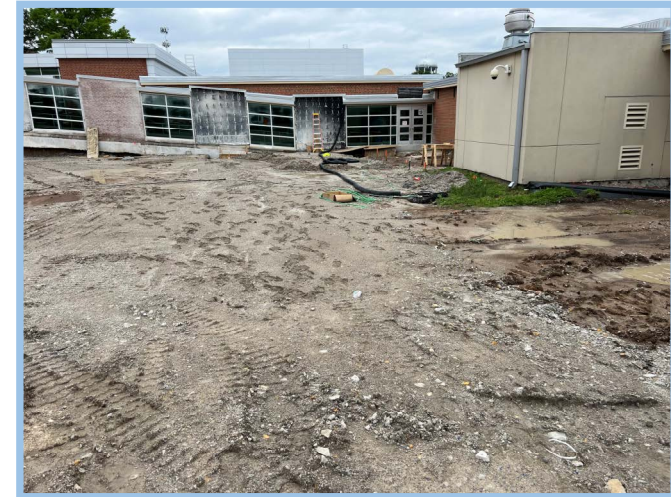
Temporarily Reroute Roof Drain
