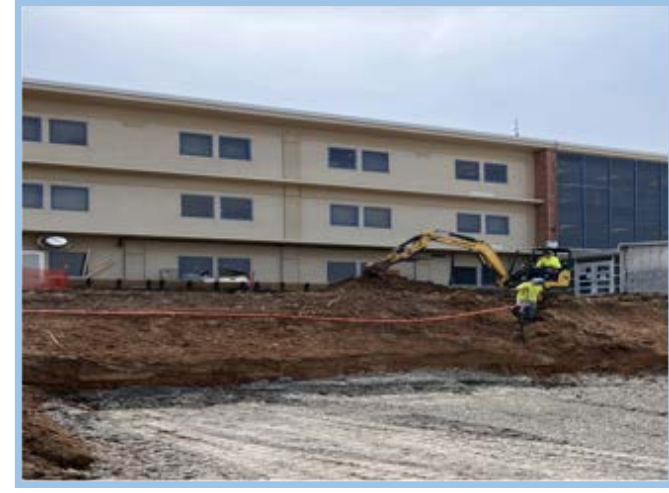
Relocate Existing Fiber Line
