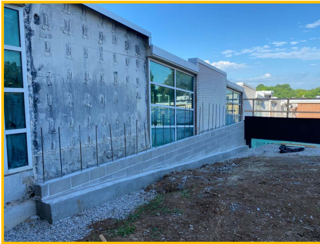
New Footing & Block Retaining Wall
