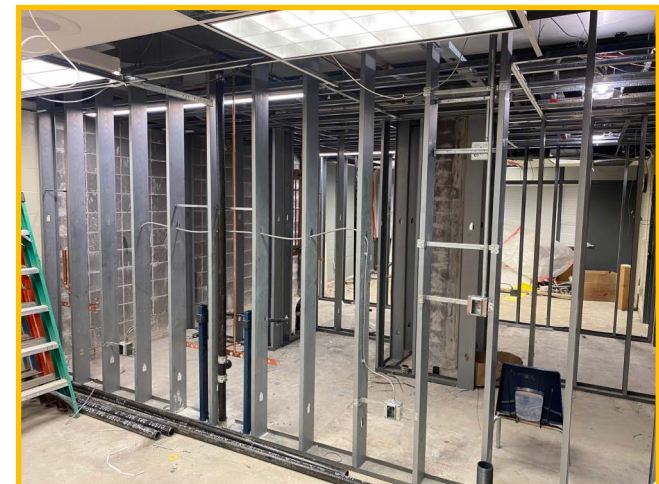
Level 1 Office/Restroom Framing
