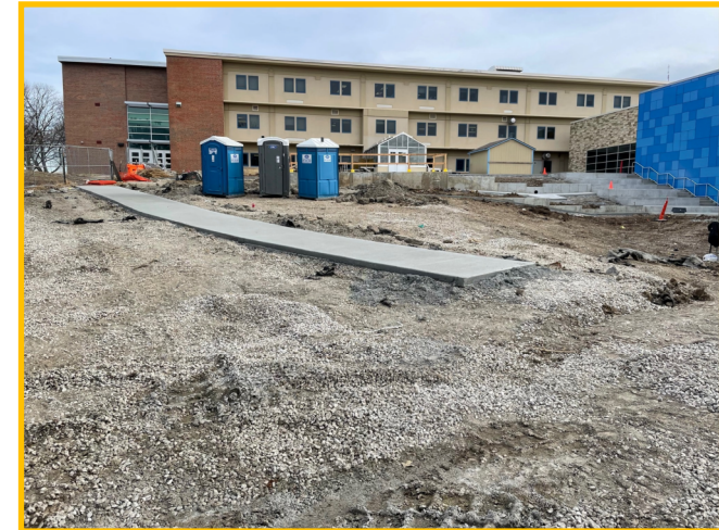
New Sidewalk Block Out to Fine Grade
