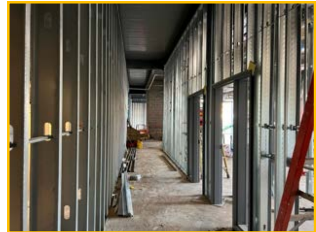
Level 3 Interior Framing
