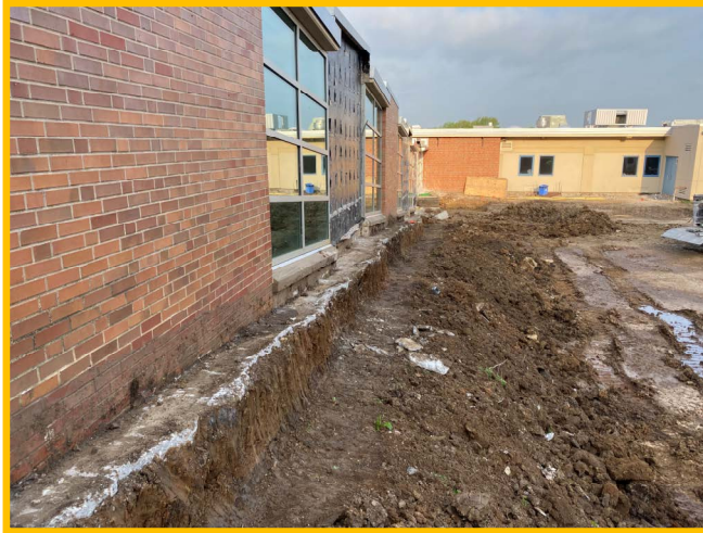
Saw Cut Existing Footing/Haunch
