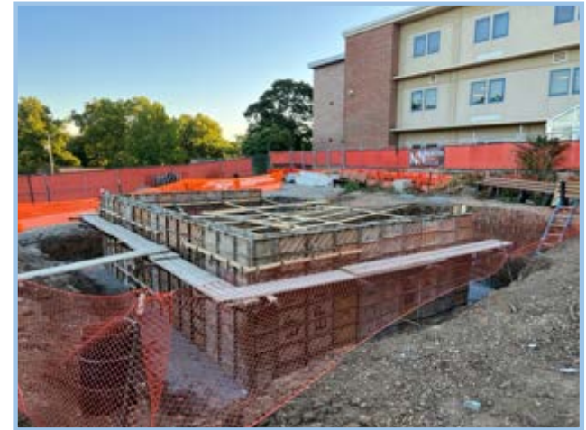
Courtyard CIP Retaining Walls
