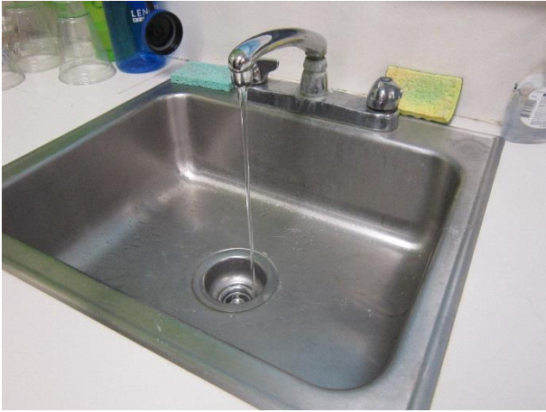
Hot water supply in classrooms has low pressure.
