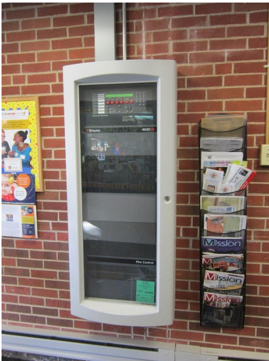
Updated fire alarm system Capable of expansion to mass notification.
