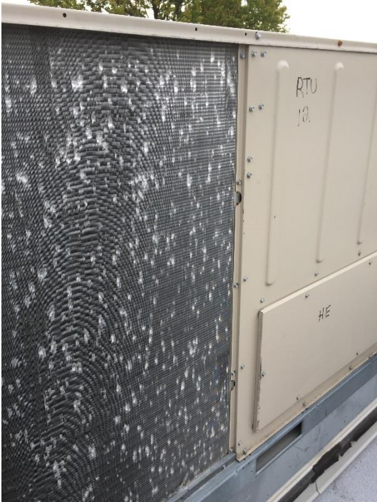
Damaged condenser coil fins.
