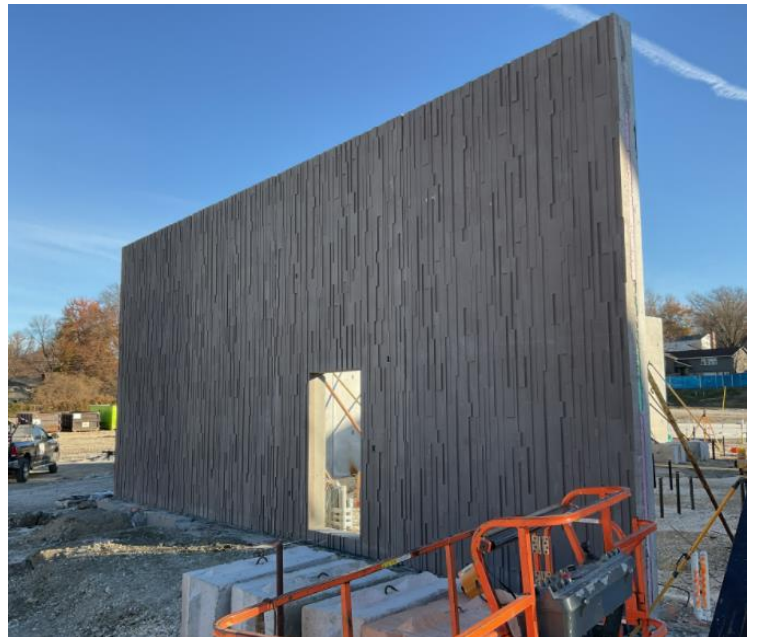
Exterior Precast Formliner
