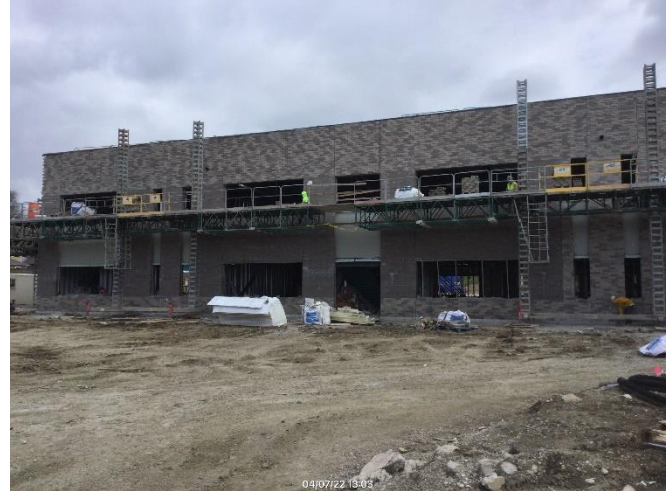
Area D brick masonry installation
