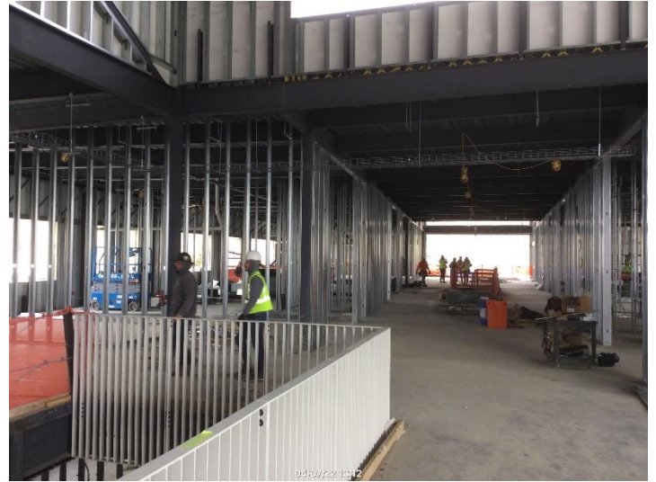
2 nd floor Interior Framing
