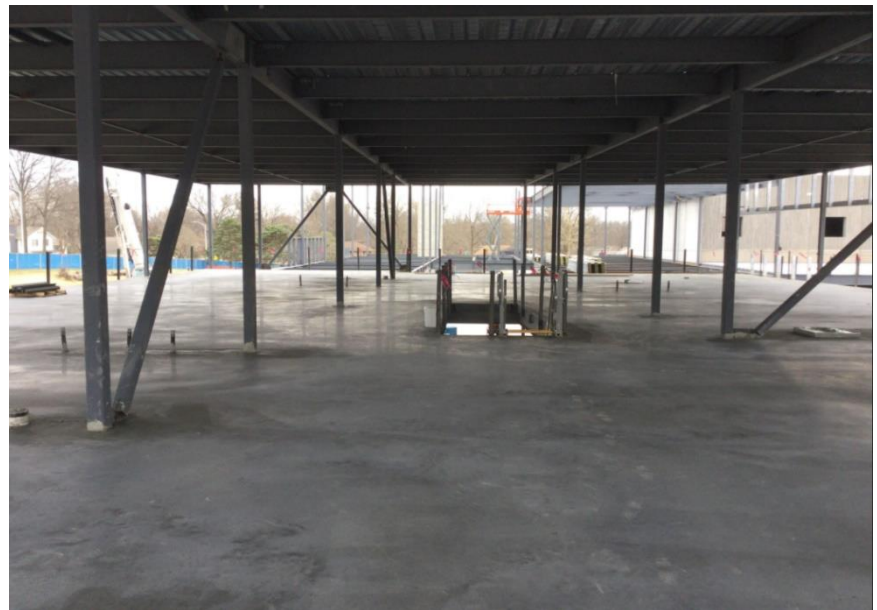
Area D Slab-on-Deck
