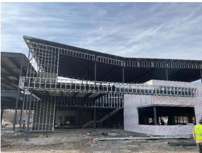
Area B Front Exterior Framing
