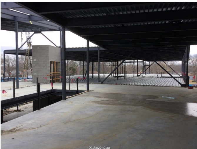
Area B Slab-on-Deck
