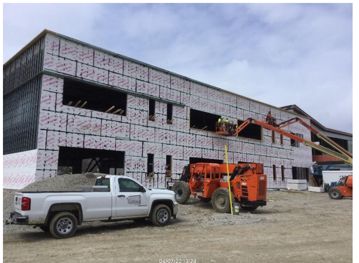
Exterior sheathing at Area A
