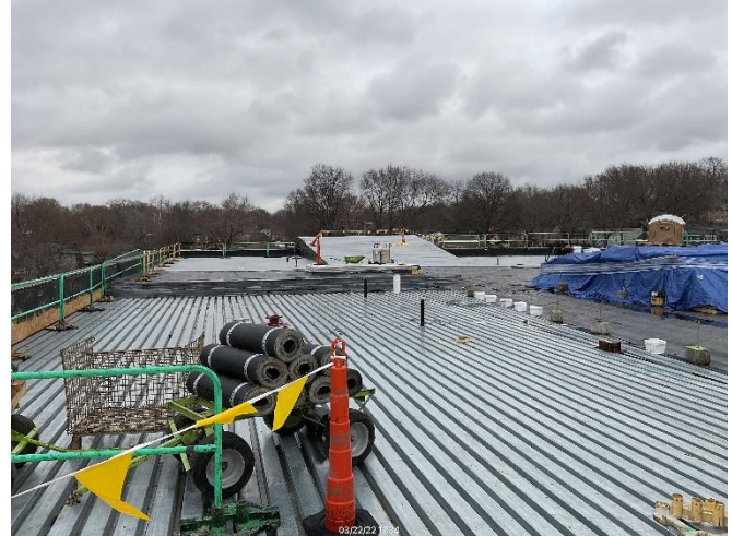
Area D Steel Roof Decking
