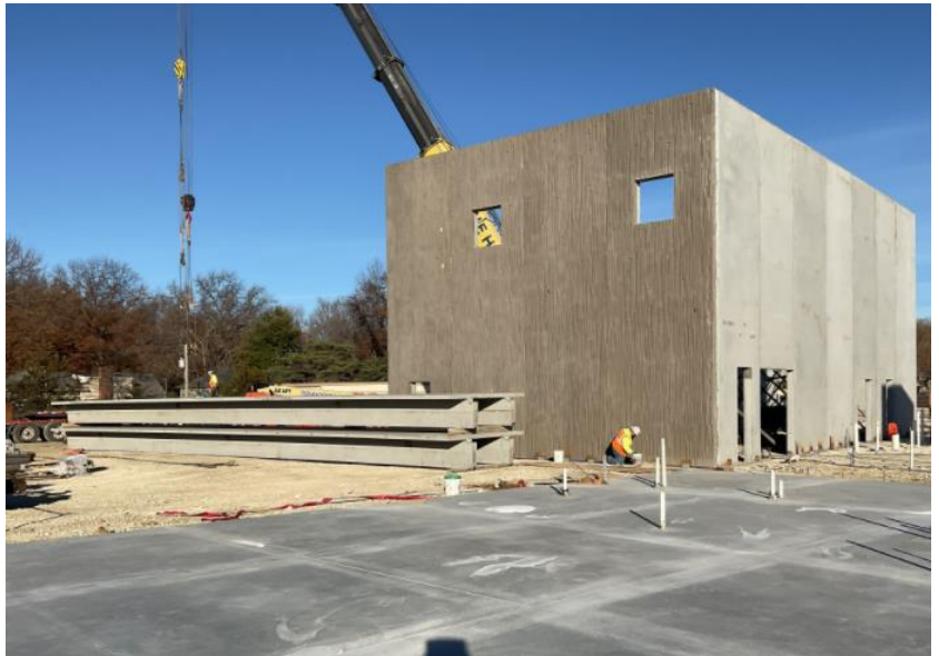
Gym Walls and Double T Roof Structure
