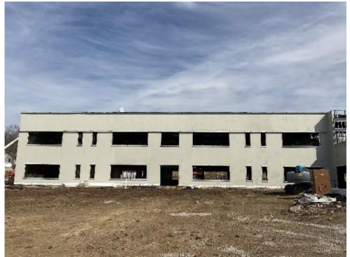
Area D Exterior Spray Air Barrier
