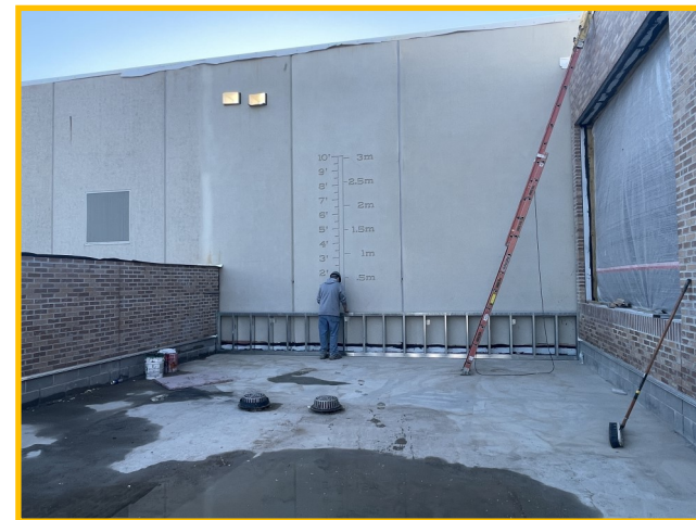
Parapet framing at Outdoor Classroom
