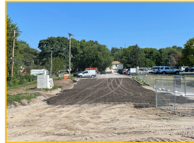
Construction Entrance Asphalt Prep.
