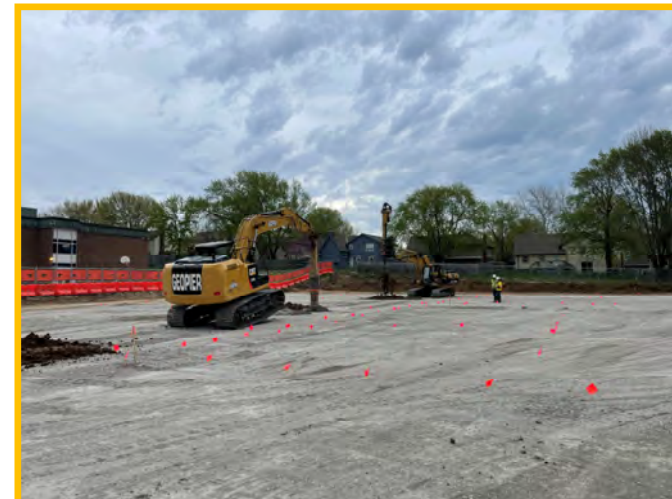
Completed Aggregate Piers
