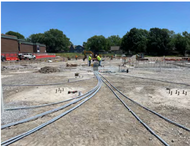
Plumbing & Electrical Underground
