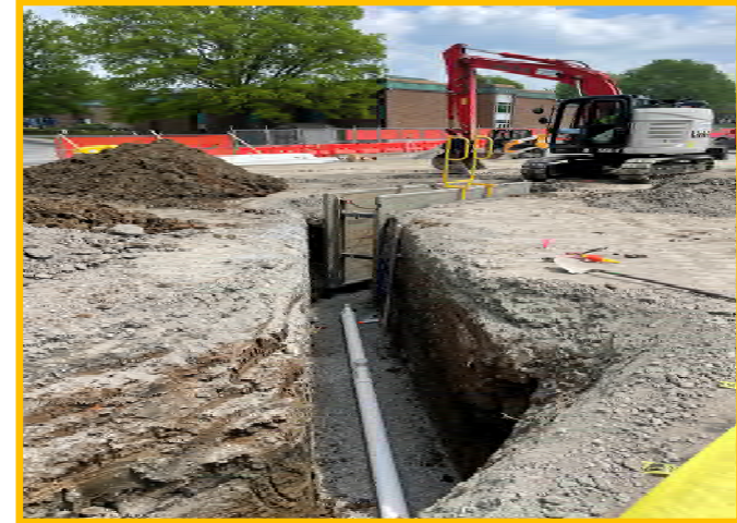
Install Plumbing Underground
