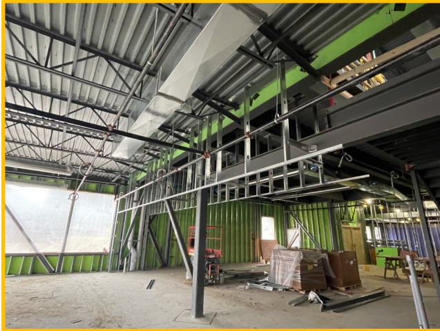
Soffit framing in Area A
