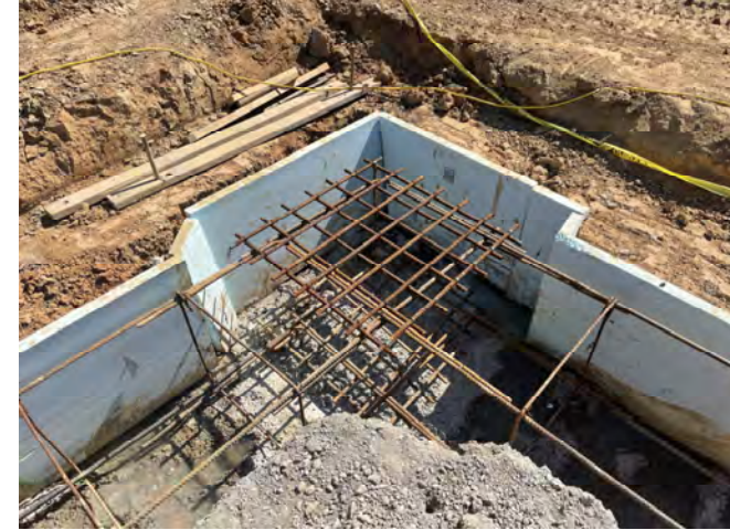
Continued Footing Formwork & Prep
