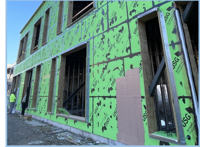
Detailing Prep Before Air Barrier
