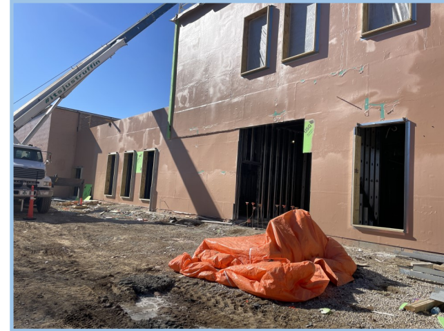
East Air Barrier Install
