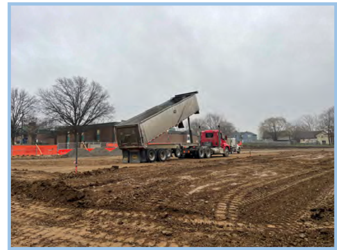
Imported Material For Building Pad
