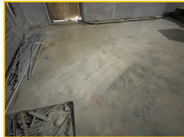
Gym Slab Prep for Wood Floor
