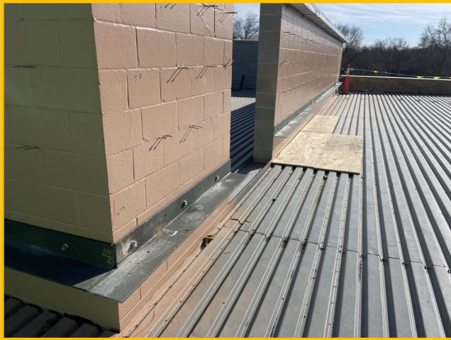
Steel Lintel for Masonry Set
