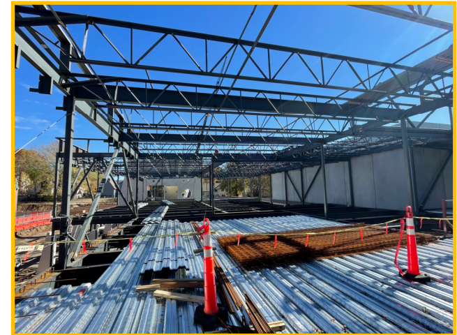
Sequence 2 Decking Install
