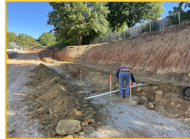
Retaining Wall Layout & Staking
