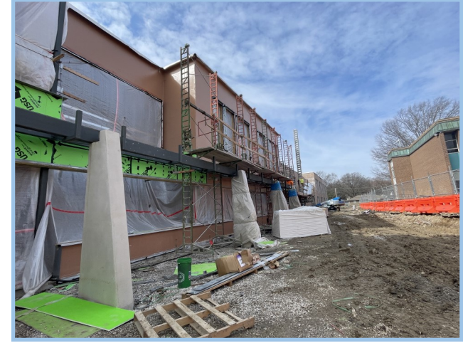
Masonry at Front Canopy
