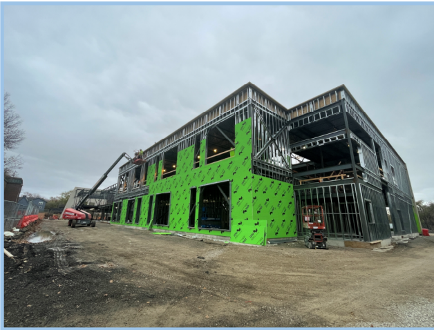
Area B Exterior Framing & Sheathing
