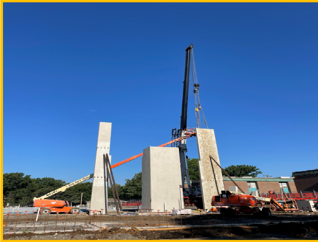
Elevator Core Precast
