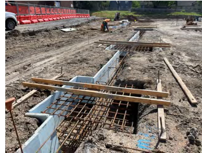
Continued Footing Formwork & Prep
