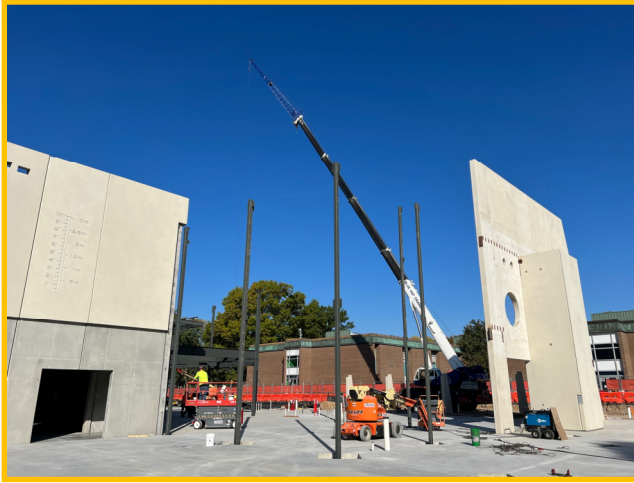
Area A Steel Erection
