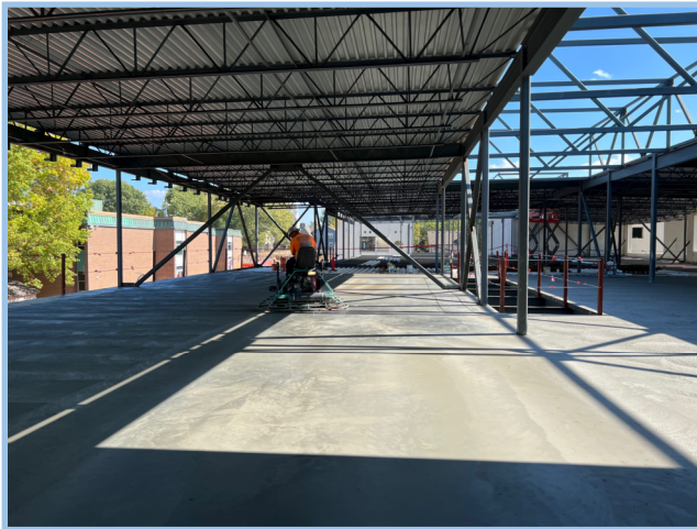
Area B Slab On Deck
