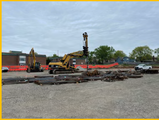
Footing Reinforcement Delivery
