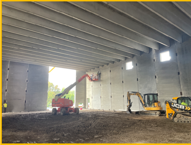
Finalizing Welding Connections
