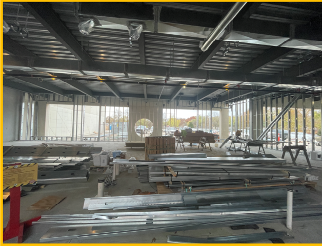
Area A Interior Stud Framing
