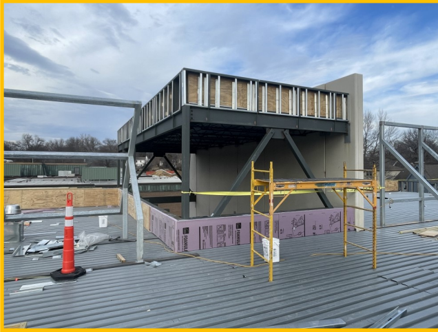
Area A Parapet Blocking
