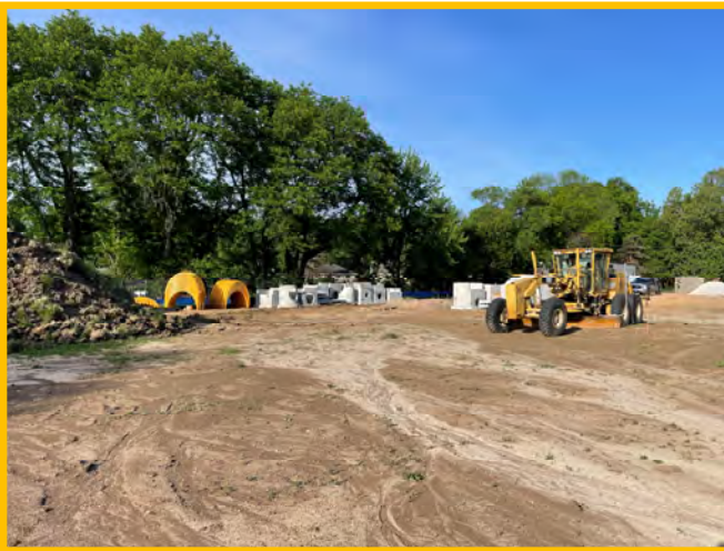
Prep Water Detention Material
