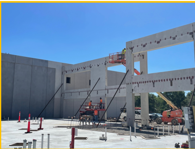
Finalizing Welding Connections
