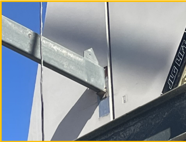
Area A Steel and Precast Connection
