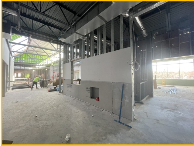
Framing & Drywall in Area B
