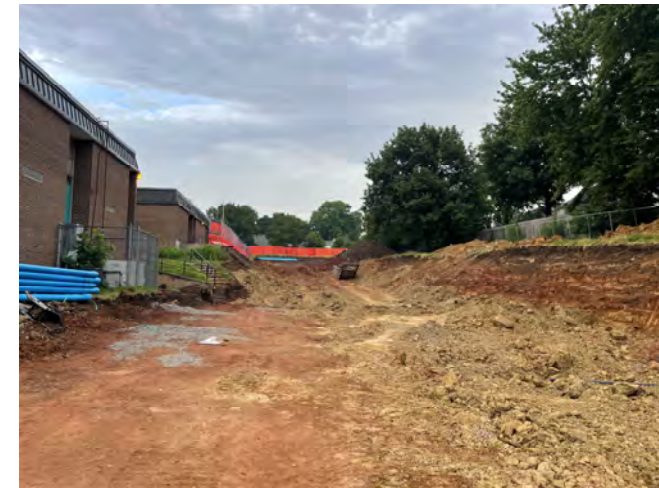
East Side Backfilled to Grade
