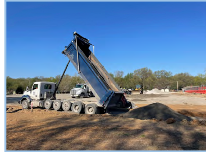
Raising Grade At Laydown Area
