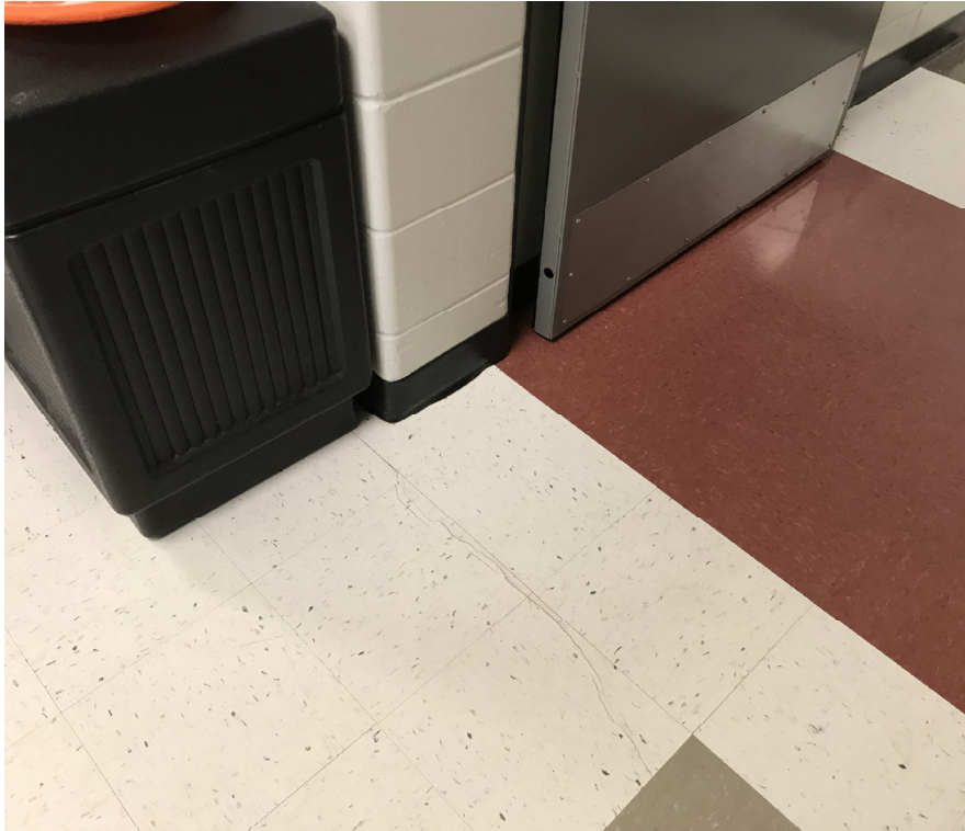
Cracking in the vinyl tile floor.
