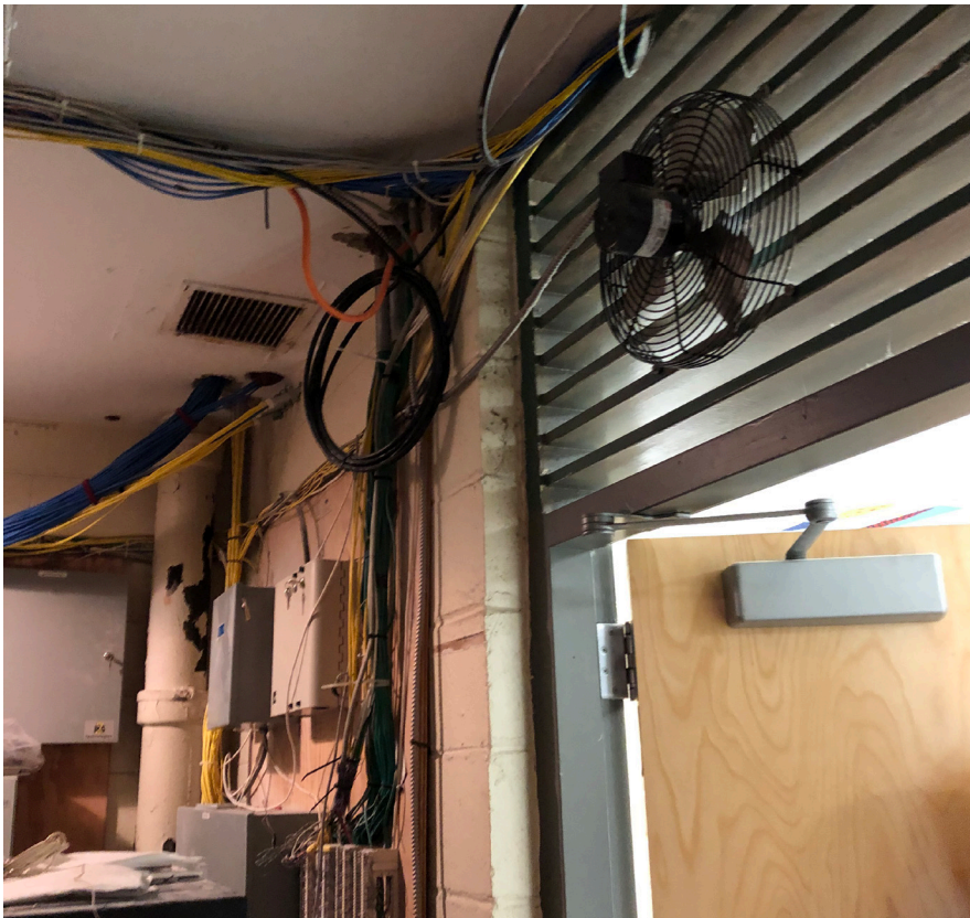
No dedicated cooling for data room, only louver above door
