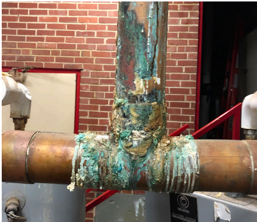
Corrosion on domestic water piping
