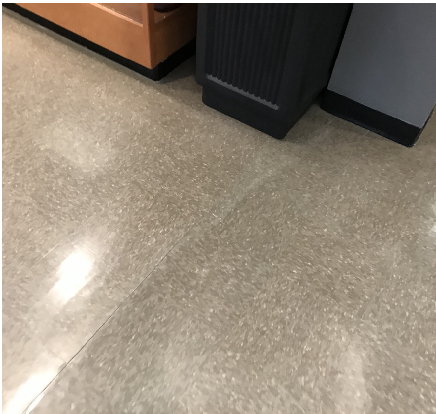
Crack in floor slab created telegraphing through the floor tile are this location in the main hallway.
