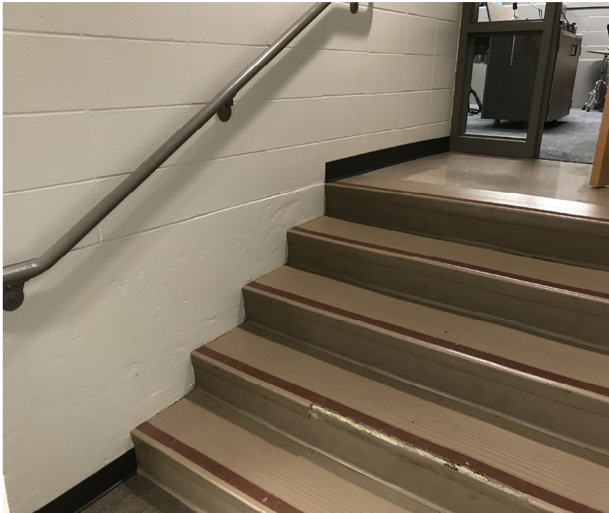
Stair nosings and tread are worn and need replacement.
