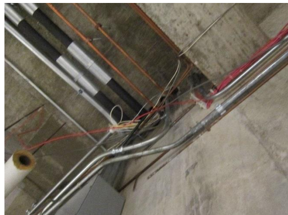
Uninsulated piping & cabling supported on pipes.
