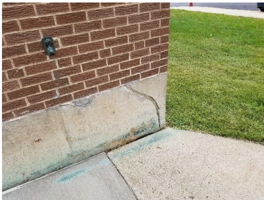
Damaged foundation wall
