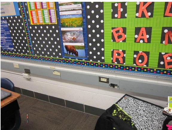
Surface raceway for outlets, devices damaged.
