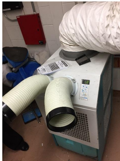
Portable air-conditioner for data rack.
