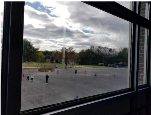
Storefront glass – loss of seal
