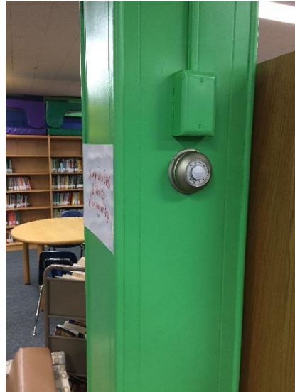
No humidistat for humidity control.
