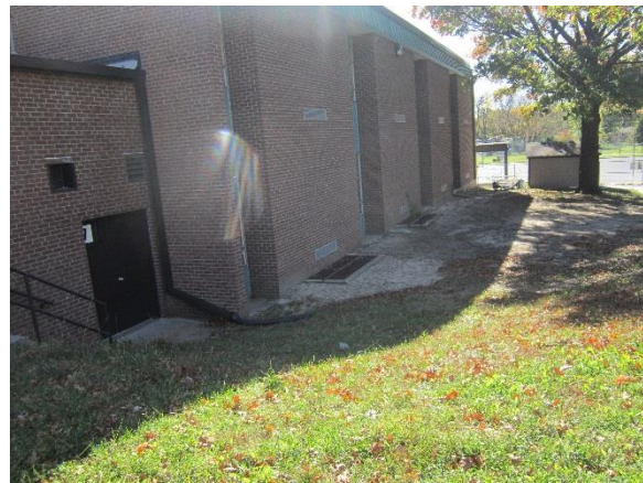
Storm shelter ventilation intakes located below grade.
