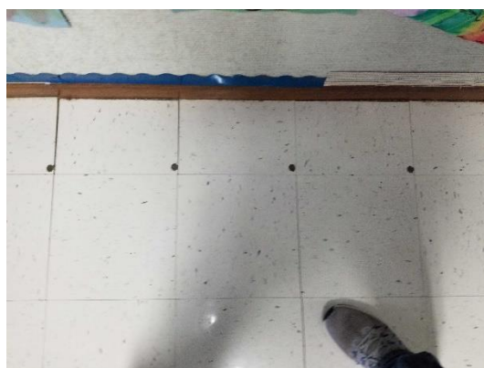
Mudjacking holes in corridor
