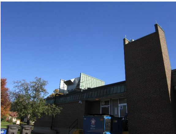
Rooftop unit with limited clearance to roof edge.
