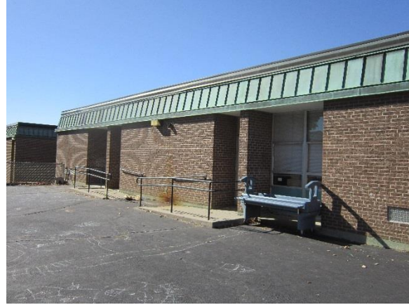
Roof drainage directly on sidewalk & discolored lightly.
