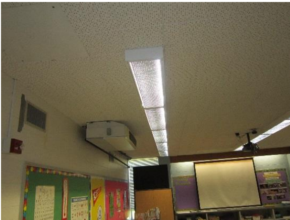
HVAC unit & piping exposed in classroom.
