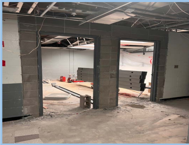
Level 1 New Openings Infill
