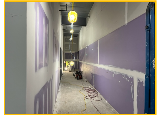
Level 3 Drywall Tape & Finish
