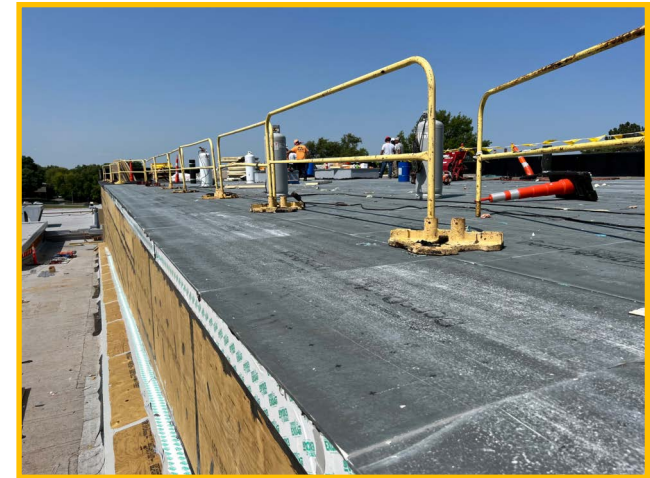
Mod Bit Roofing Install
