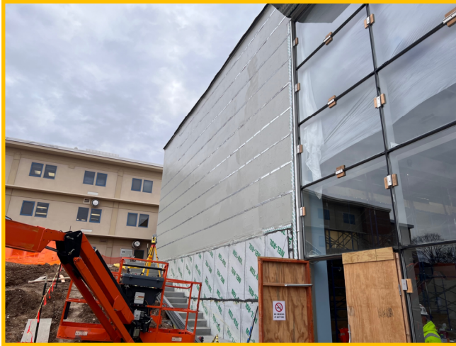
North Elevation Phenolic Panel
