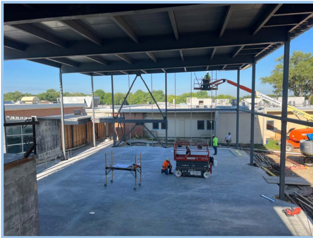
Level 2 Exterior Framing
