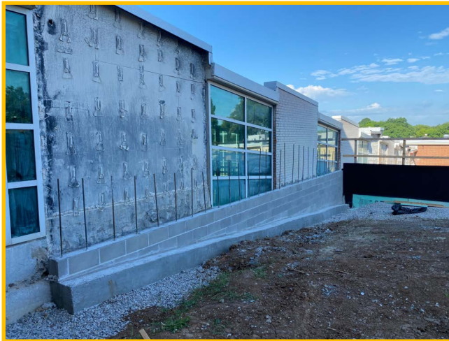
New Footing & Block Retaining Wall
