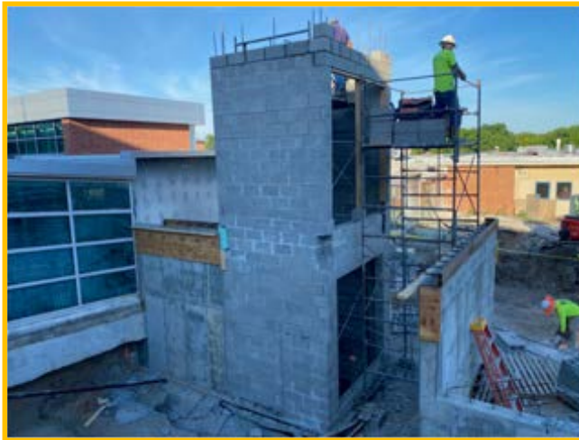
Elevator Shaft
