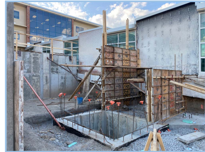
Pour CIP Walls South Of Elevator Pit
