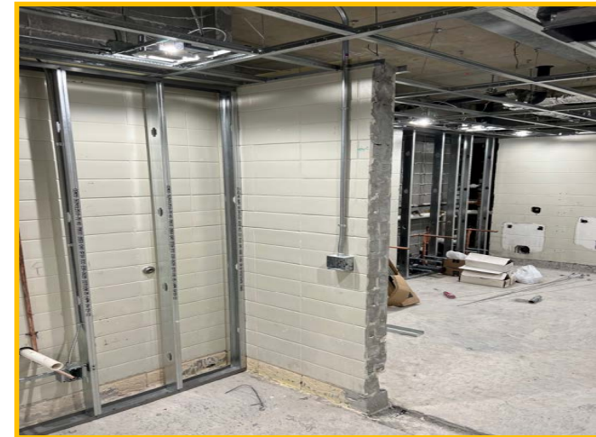
Level 4 Framing & In-Wall
