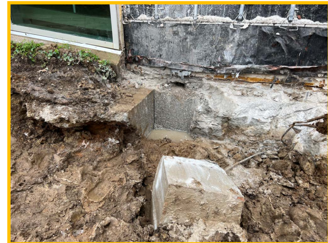
Structurally Upgrade Existing Footing
