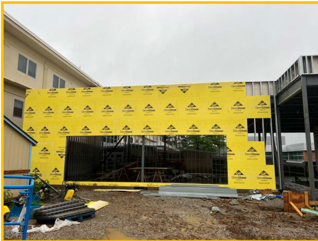
Exterior Framing and Sheathing
