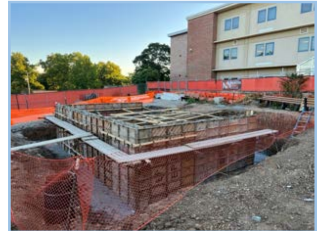
Courtyard CIP Retaining Walls
