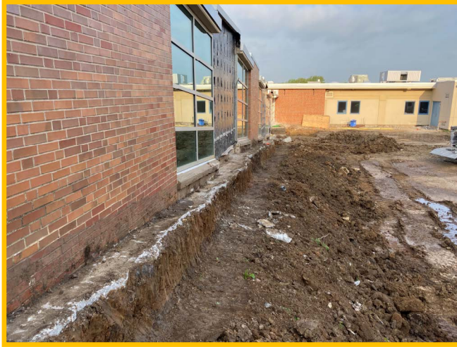
Saw Cut Existing Footing/Haunch
