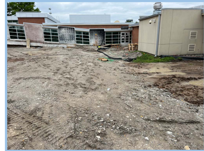
Temporarily Reroute Roof Drain
