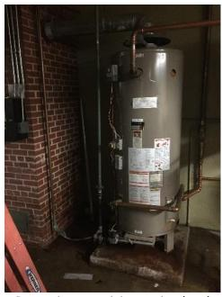
Domestic water piping not insulated In mechanical room.
