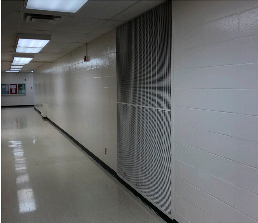
Mechanical return air grille for AHU
