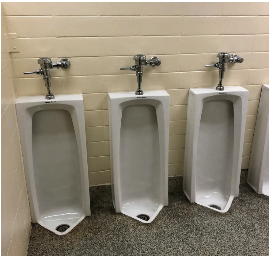
Plumbing fixtures not upgraded
