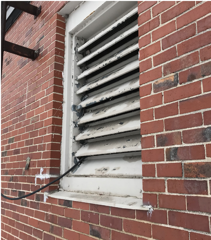
Refinish louvers and tuck point brick joints.
