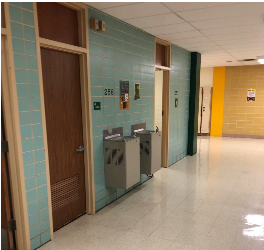
Water cooler not ADA and no bottle filler
