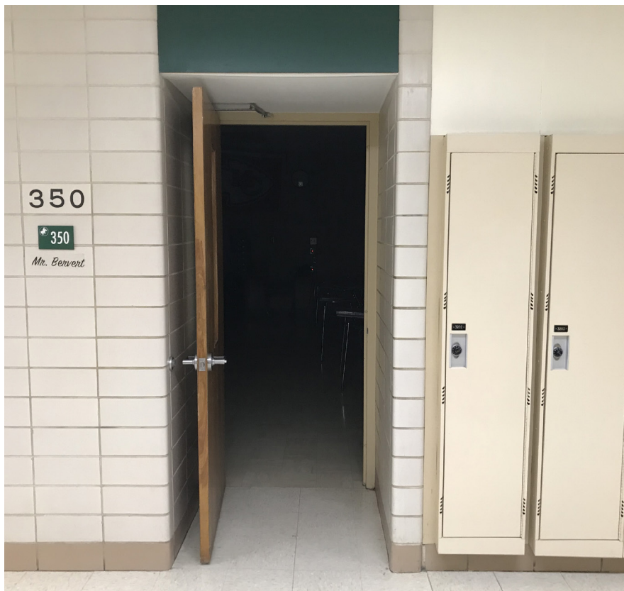
Classroom access in the older parts of the building may not comply with current door clearance requirements (accessibility requirements).
