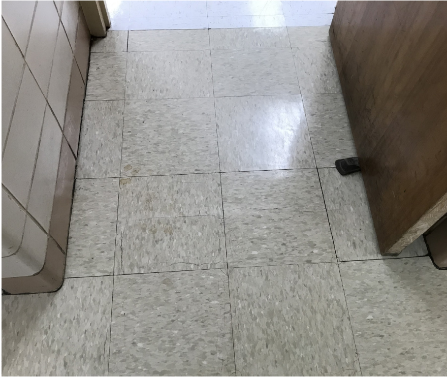
Floor tile is cracking at the original building portion.
