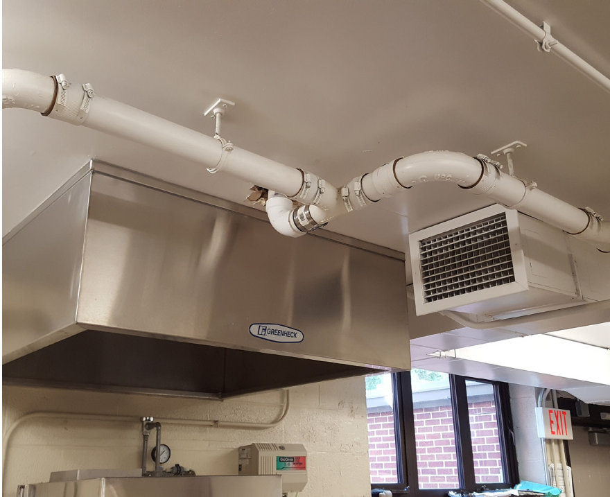
Sanitary vent piping near kitchen dishwasher
