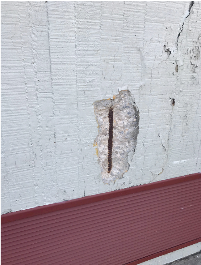
Concrete surface deterioration due to moisture issues.
