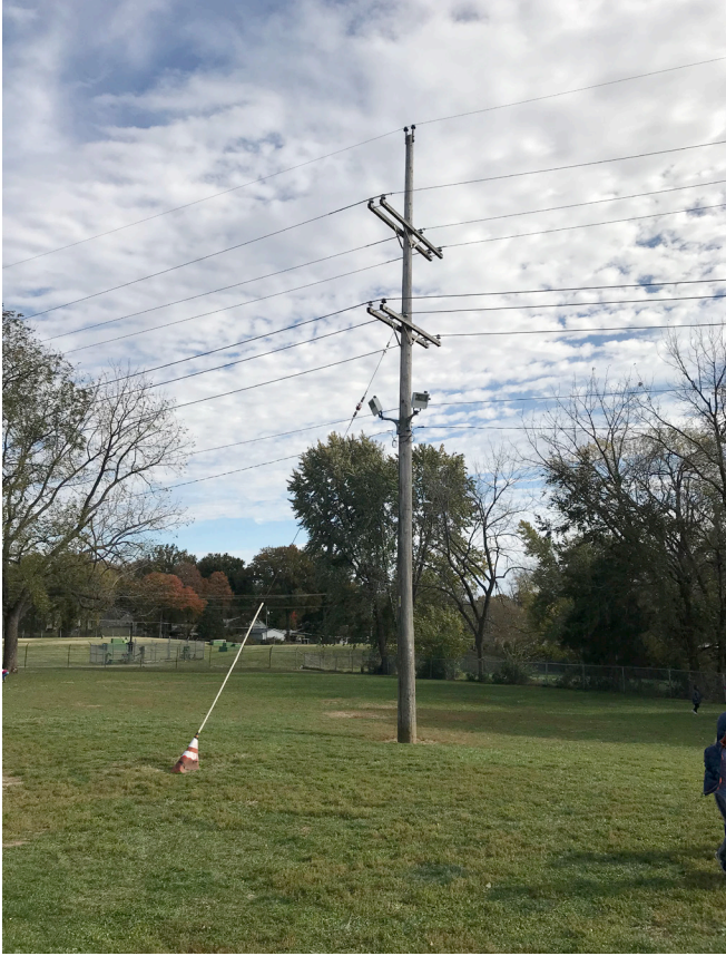
Overhead powerlines running through the playground areas. Guy wires are a tripping hazard.
