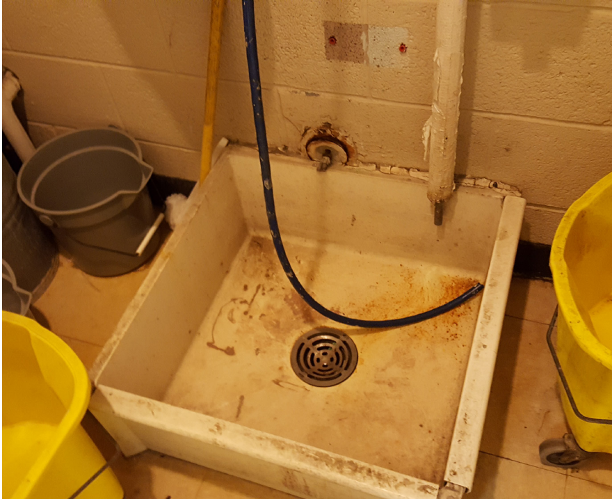
Mop sink deteriorated recommend replacement
