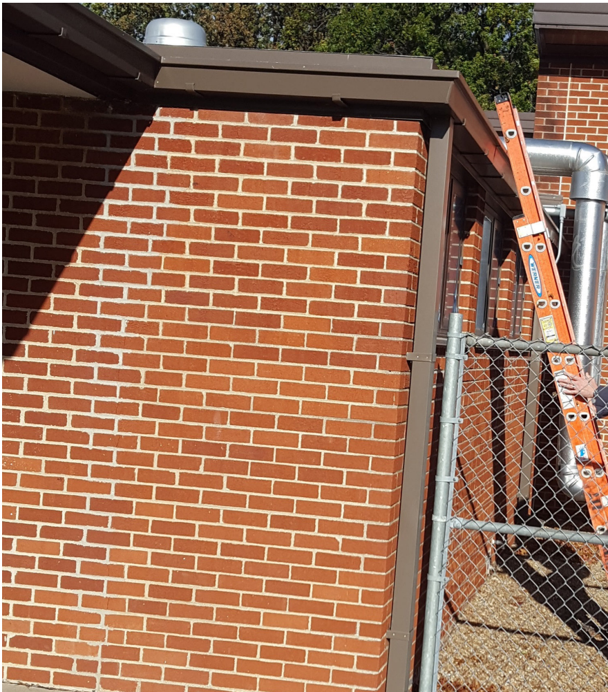
Roof Access is not permanent
