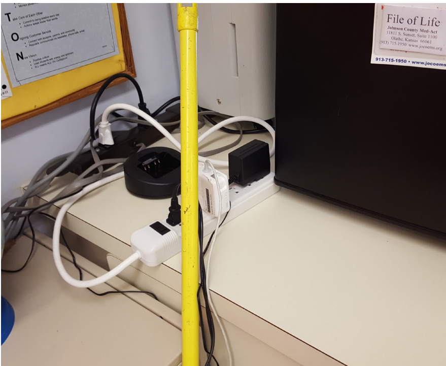
Insufficient electrical outlet quantities
