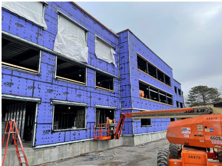
Air Barrier Install
