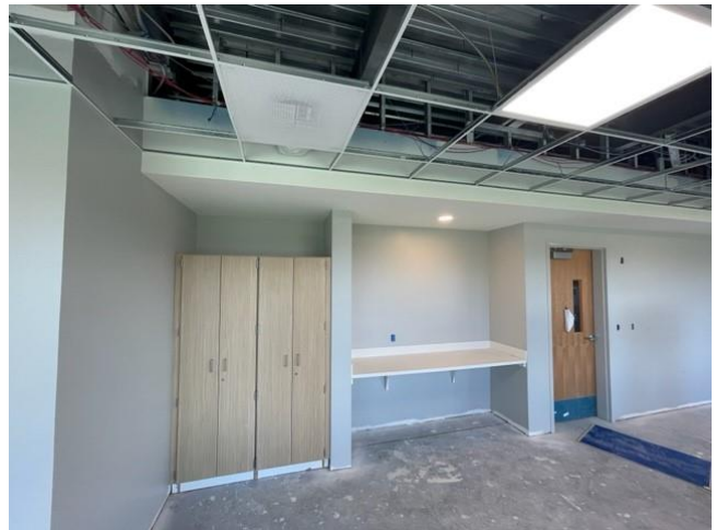
Ceiling Grid and Counter Tops Installed
