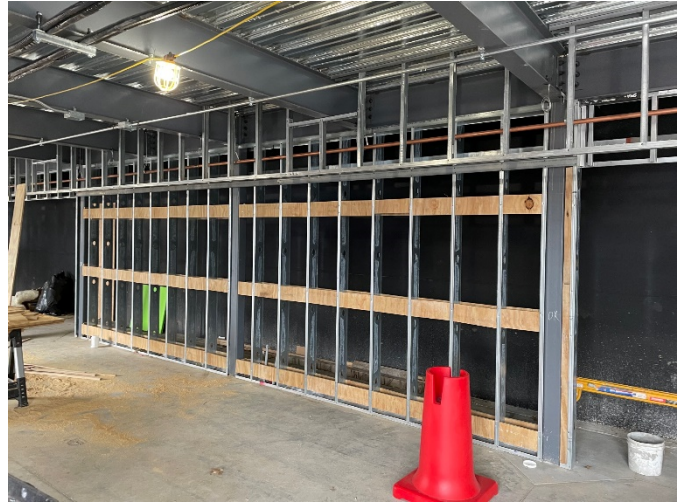
Blocking for Rulon Wall
